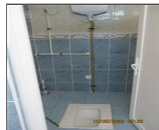
Photo of the sanitary facilities TOILET .JPG
